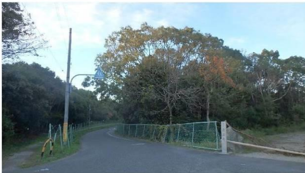
樹木剪定：④ (施工前)
